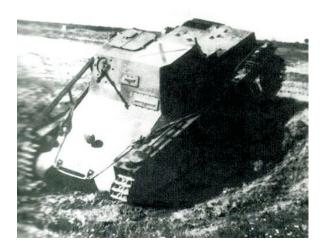
This kit represents the rare early version of the kl.Pz.Bf.Wg.I. Ausf.B, which saw action during Spanish Civil War. It differs from the later mass-produced version of the kl.Pz.Bf.Wq.I. Ausf.B - the MG turret has no ball mount, and the upper hatch is flat, while the later common type has a commander's tower.
